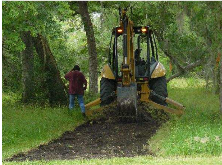
Removing Topsoil.
