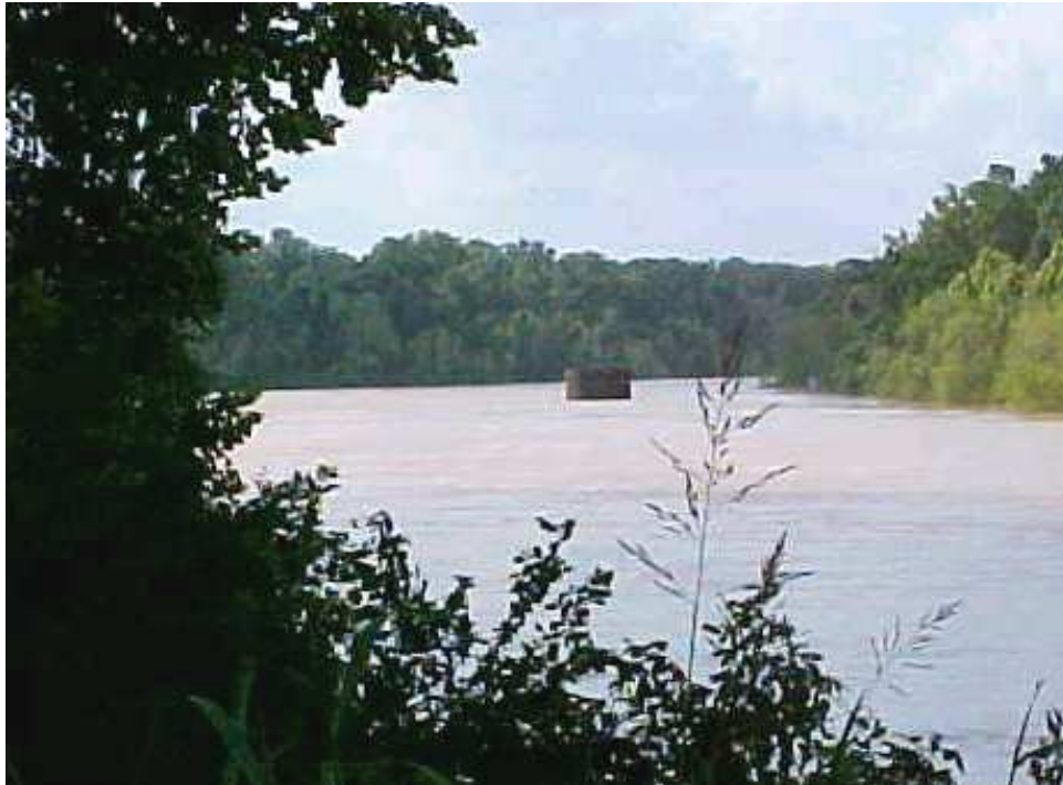
Abandoned Bridge Pier, seen from Brazoria Bridge Photo: Neal McLain
