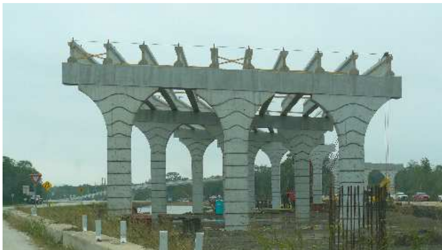
SH332/FM521 Highway Bridge Under Construction, 2008 Photo: Neal McLain
